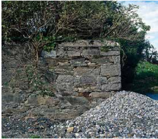
Figure 16.40 Image of traditional stone wall at Devoy Barracks, Co. Kildare
