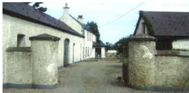
Figure 16.17 Linear farm complex, Caragh Road, Naas.
