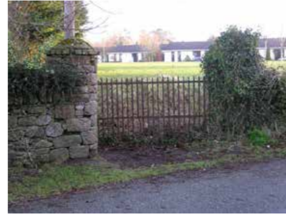
Figure 16.42 Stone wall, pillars and gate, Naas
